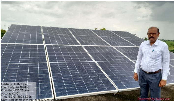
Solar Panels are installed in college
